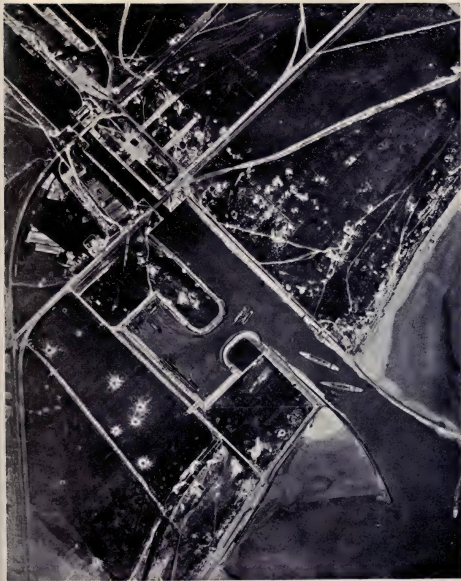
AERIAL PHOTOGRAPH SHOWING THE POSITION OF THE BLOCK SHIPS AT ZEFBRUGGE
