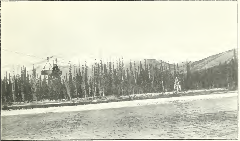
Cable station on Athabasca River at Jasper, Alberta.
